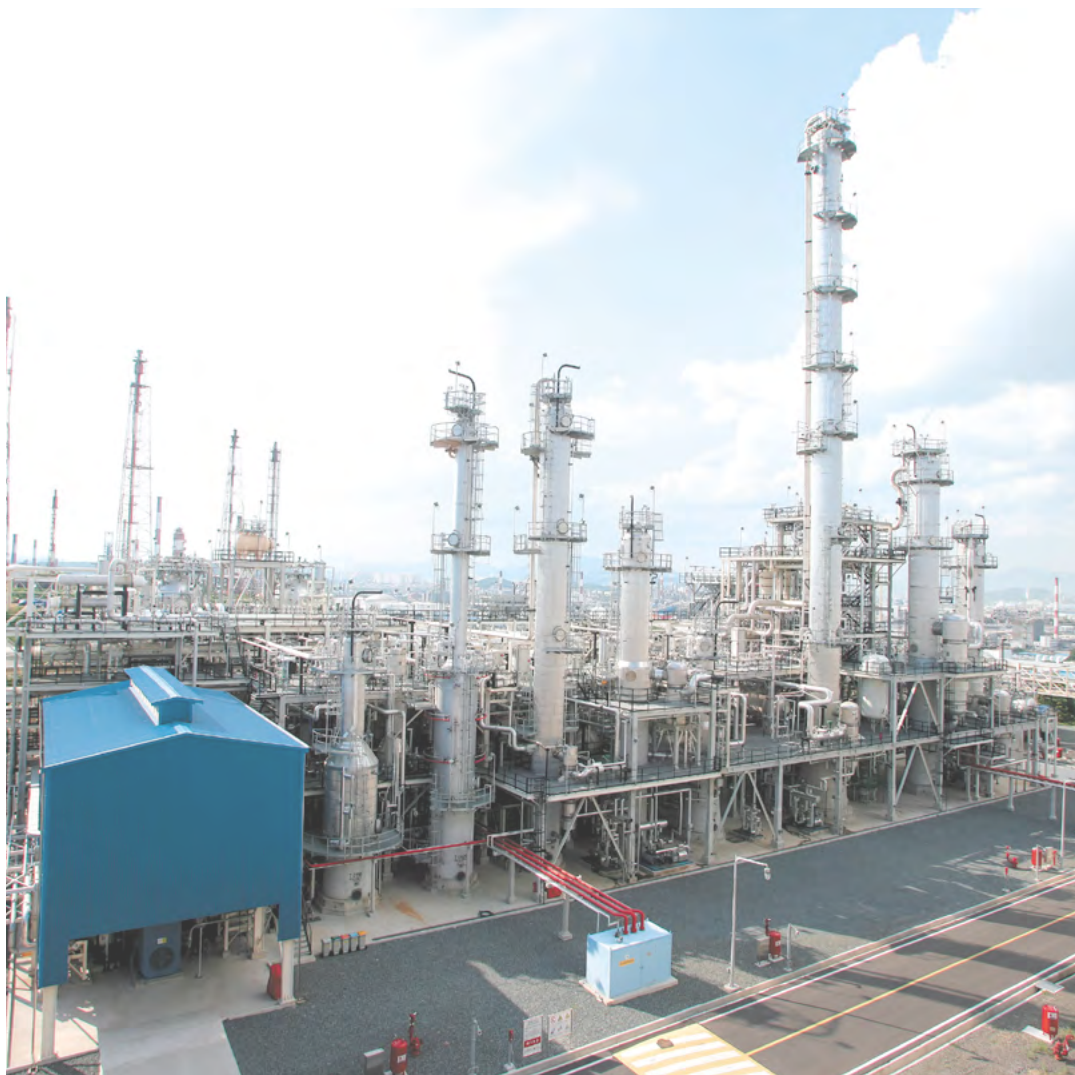
HPPO plants are typically built right next door to a hydrogen peroxide plant, so that the oxidant can be piped directly 'over the fence' for the clean, green production of propylene oxide.
