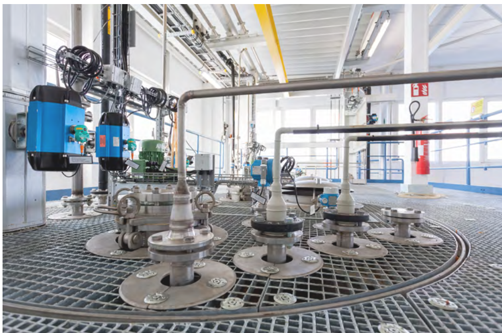
A wastewater treatment plant that uses Eisenmann's proprietary, two-reactor Fenton's reagent-based process called Fentox.
