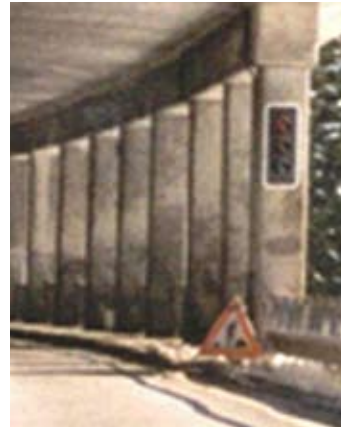
Tests performed on steel reinforced columns (pictured left) at the entrance of the gallery of Cianca Presella located on the Swiss Highway A13
