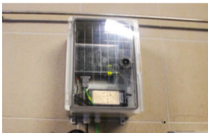
Gateway Siemens IoT2050 equipped with WiFi sends data to Siemens IoT cloud
